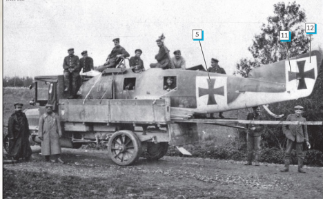
This photo is believed to show the salvage of Roland C.IIa 1666/16, if true, this is one of the very 1st late production batch Roland built C.IIa with aileron control rods running through the top wing ordered in April 1916 (numbers 1664/16 to 1699/16). Note the aileron control rods (5) under the top wing root.
